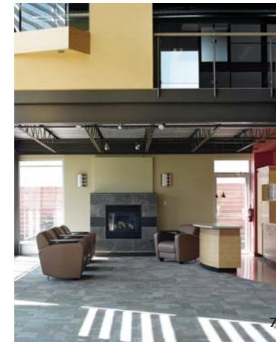
THE EXPOSED STEEL STRUCTURE MINIMIZES FINISHES AND DIVERTS ATTENTION TO THE INTERFACE FLOOR COVERING. THE METAL DECK REFLECTS NATURAL LIGHT AND HAS PERFORATIONS FOR SOUND DAMPENING [7].
