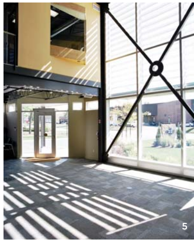
LIGHT STREAMING THROUGH THE LARGE SOUTH WINDOW, BRACED FOR LATERAL RIGIDITY, REDUCES HEATING REQUIREMENTS AND CREATES A VIBRANT INDOOR ENVIRONMENT [5]. THE VIEW OPPOSITE PHOTO 5, NOTE HOW THE INTERIOR OFFICE WINDOW ANGLES TO CATCH THE NATURAL LIGHT [6].
